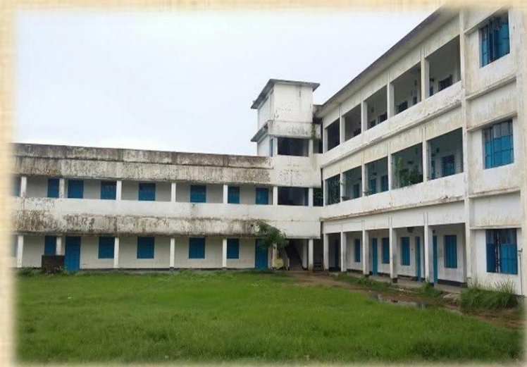
School Old Building
