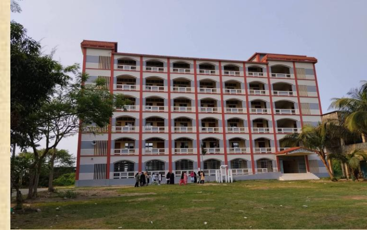
School New Building
